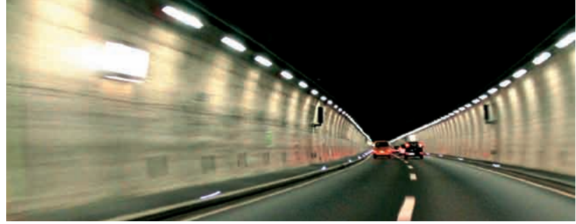
Left: GSM-R network for Beijing and Tianjin railway stations, which serves the fastest stretch of rail (speeds of up to 350 km/h) used by scheduled trains in the world. Right: Analog and digital radio for the emergency services as well as broadcasting and telepage services for all of the tunnels of the A1 and the A5, and almost blanket coverage of all of the motorway tunnels in Switzerland.
